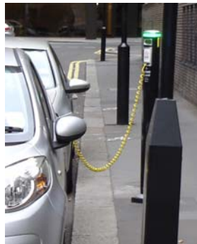
Short cable extension – minimising trip hazard
