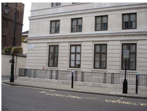
Wilton Street, Westminster Wide footway and uncluttered street. Feeder pillar in signpost housing
