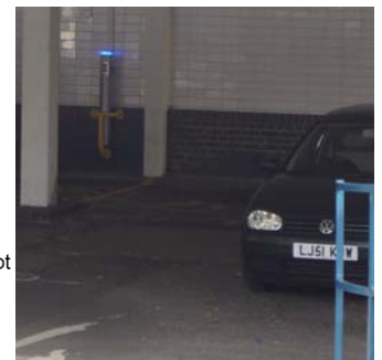
Putney Leisure Centre, Wandsworth At entrance to multi-storey car park
